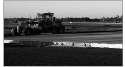
A runway construction project could be broken up into grading one year, followed by paving and final work the next.
